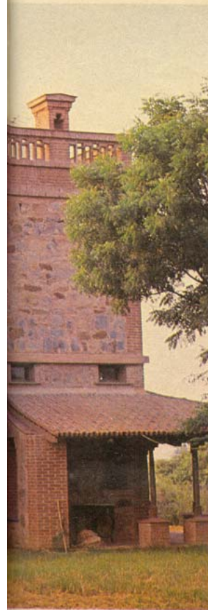
The stone house emerges as a part of the contextual landscape of Delhi
