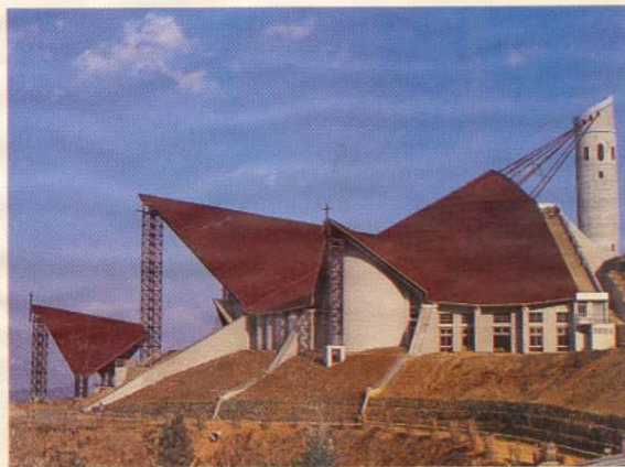
The semi-circular form of the cathedral: unconventional Right: The structural system defines the roof Far right: The reinforced concrete belfry borrows from local tradition its decorative element Previous page: Model of Kohima Cathedral
