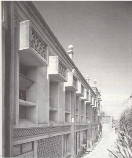
7, side elevation of the weaving mill at Kharkhana, Delhi; the projecting boxes over the windows and the jalis shade and cool the interior. 8, the flat roof on the weaving mill is used for drying cloths while the glass block rooflights and the small atrium help light the interior yet prevent the penetration of direct sunlight.
